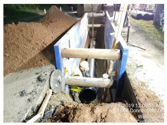
Installing 16" DIP pipe on RT. 17, Middletown near STA 106+50. Approximately 600 feet south of the intersection of Rt 17 and Talcott Ridge Drive.
